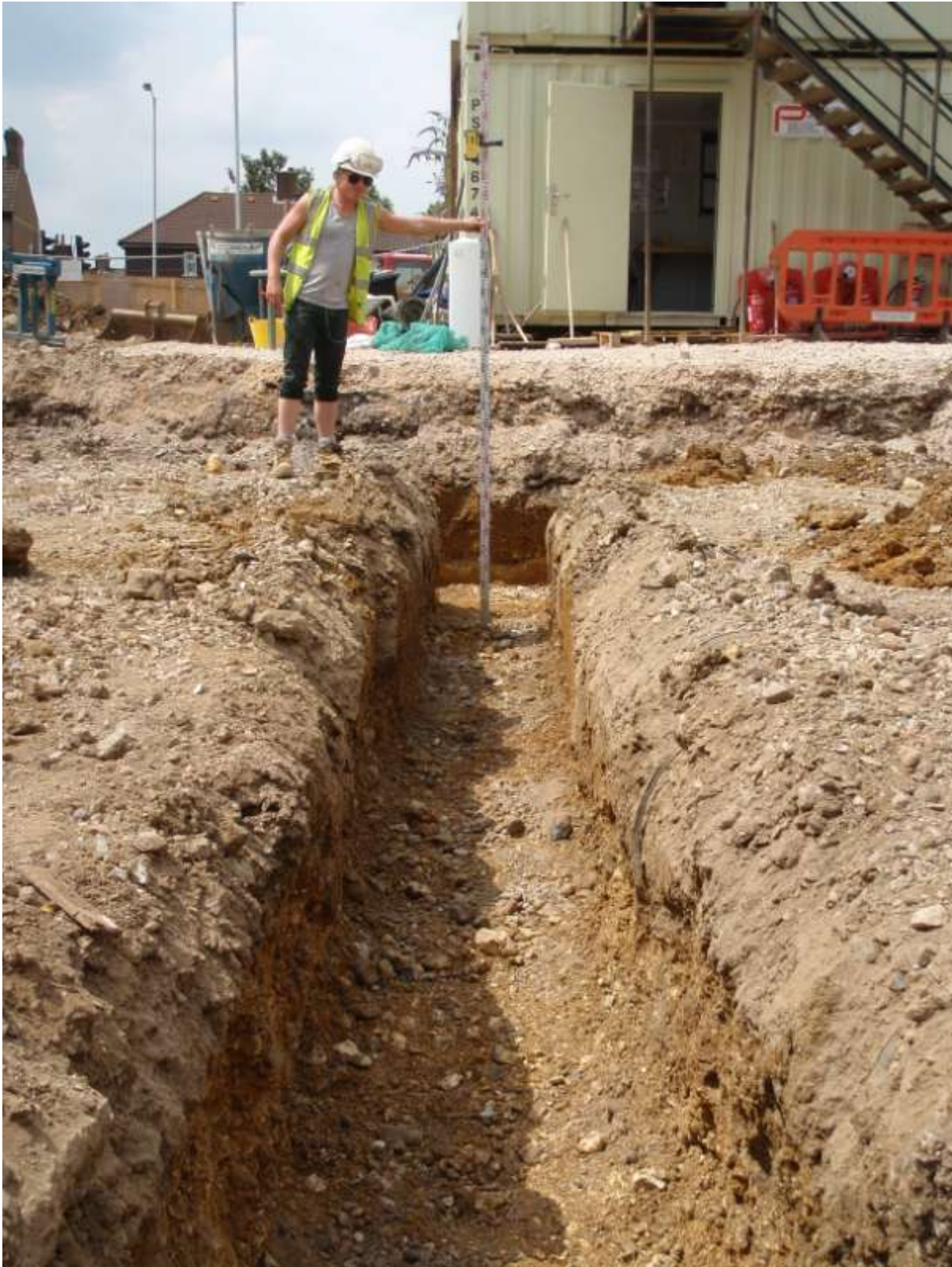
Plate 4. Foundation trenches (facing north-east)
