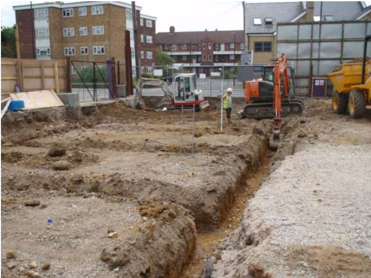
Plate 2. General view of site, facing south
